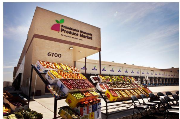
A CWSRF loan funded clean-up that led to the development of the Philadelphia Wholesale Produce Market.
