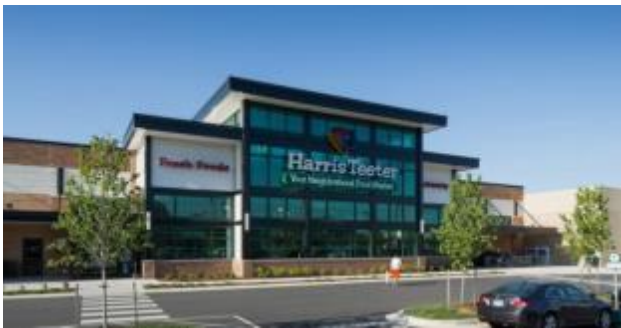
Canton Crossing, Baltimore Rebuilt a bulkhead using a CWSRF loan
