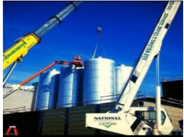
Construction of a new “destination” brewery on a brownfield in Minneapolis
