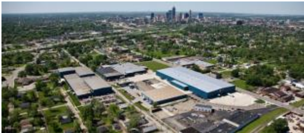
Insurance recovery was the key to re-use of this Indianapolis plant, now 500 jobs at Major Tool and Machine
