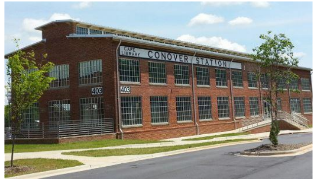
Conover Station in Conover, NC
