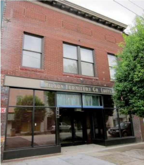
Wilson Lofts, Wilson, NC – key financing through historic tax credits
